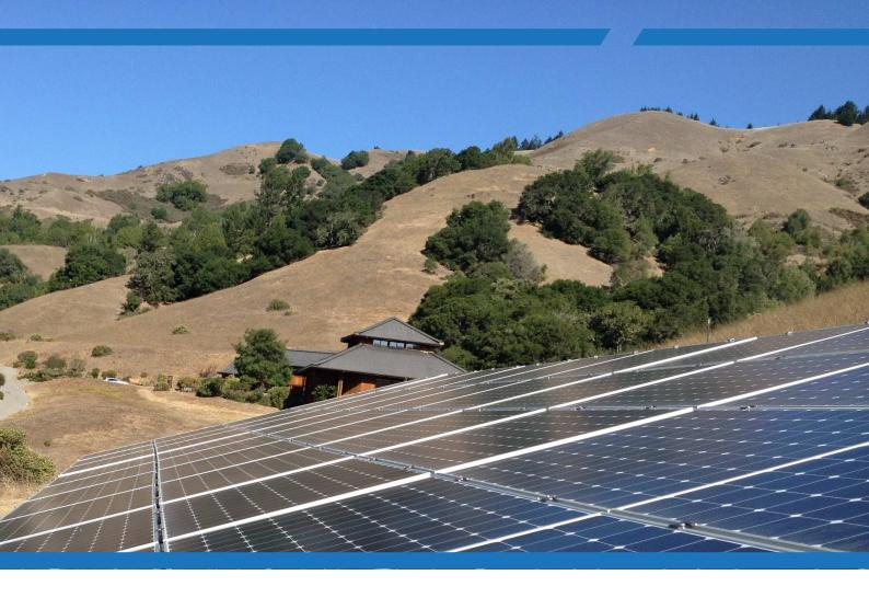
Central Distributed System, 1MW with 48 MPPTs, suitable for complex environment like uneven ground.
